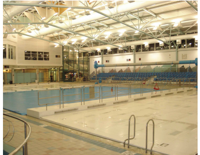
Pool covers above have contributed to a 30% reduction in energy use.
